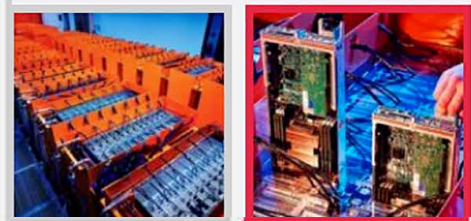
In Skybox Datacenters' liquid cooling approach (utilizing the immersion technique), dielectric fluid is cooled and circulated around hot server components. Heat exchangers are submerged with the computer equipment, meaning that no dielectric fluid ever leaves the tank. A water loop runs through the rooms and to each heat exchanger.
